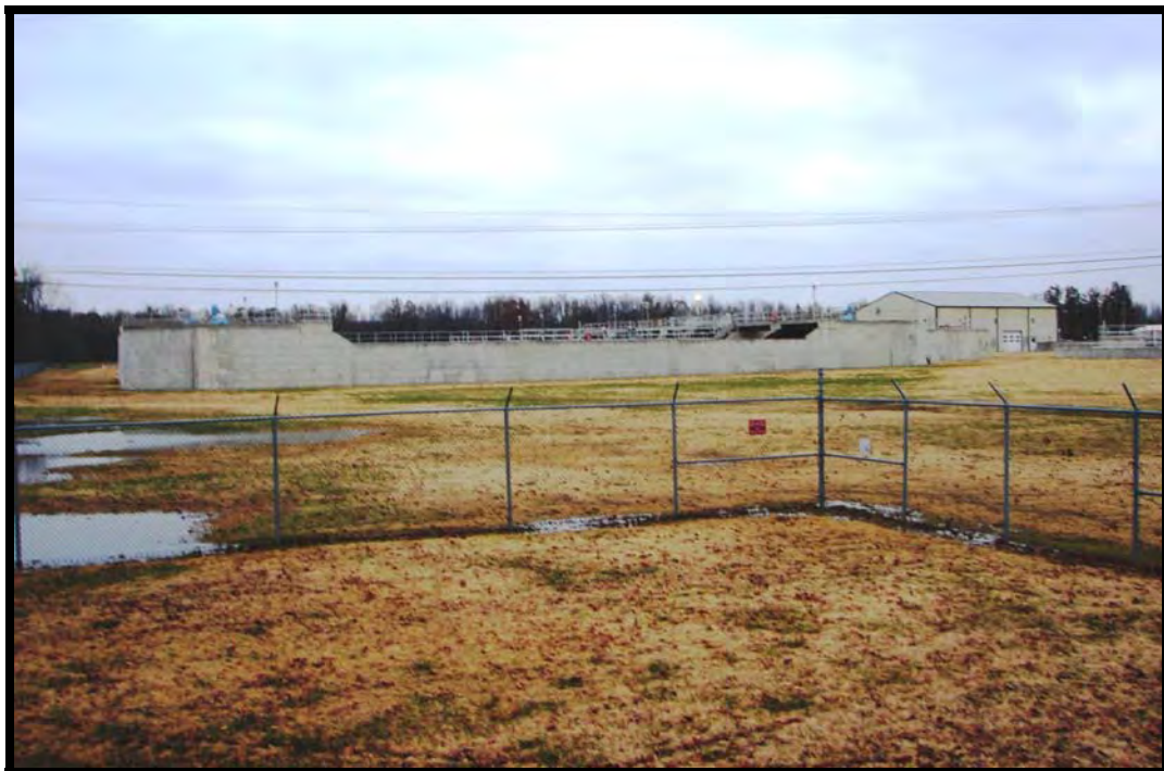
Figure 16 View of Wastewater Treatment Plant North of Alternative S1
